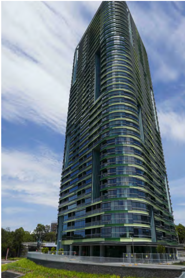
Figure 1. General view of the Opal Tower. Note the inset slots on the external faces of the building, each extending for multiple storeys (some 6 and others 10 storeys).
