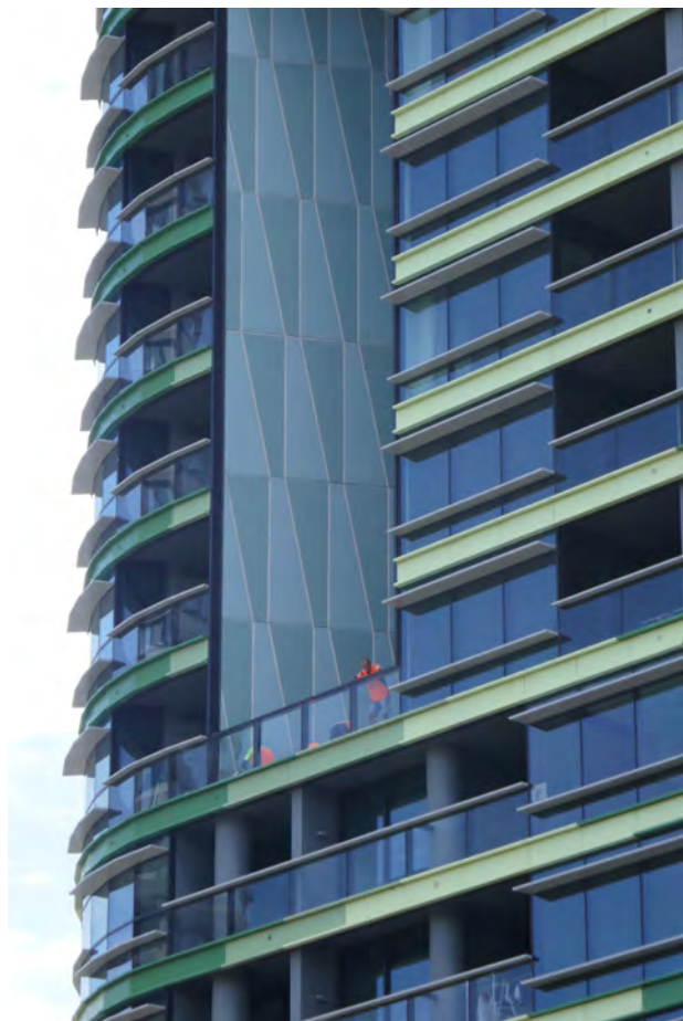
Figure 2. Close-up view of a 6 storey slot. Note the 6 panels forming the load bearing wall of the inset slot, each one storey high.
